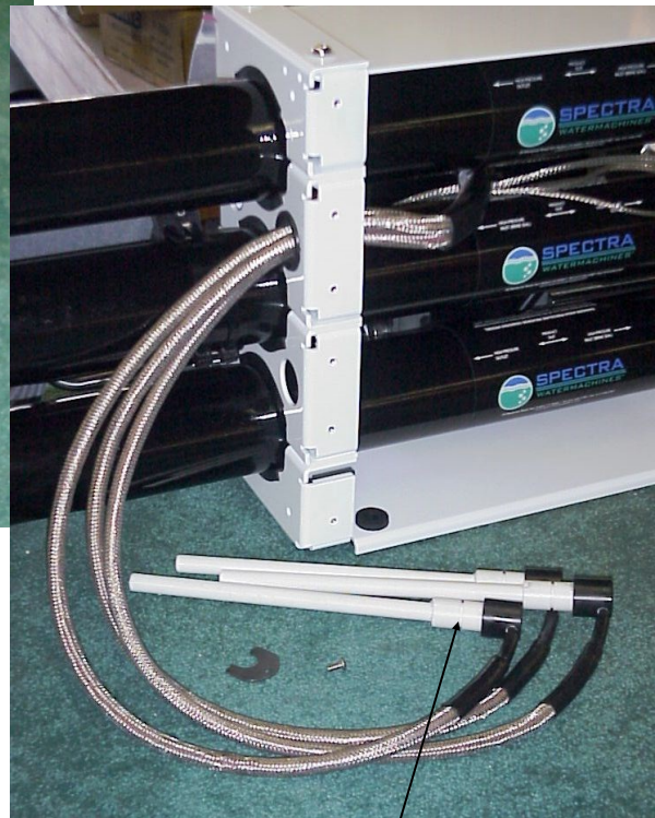
C-Clip groove in Anode
